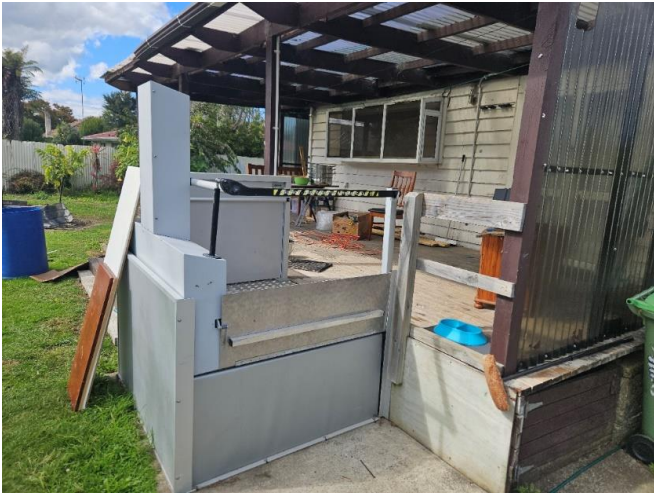
Chair lift and covered area
